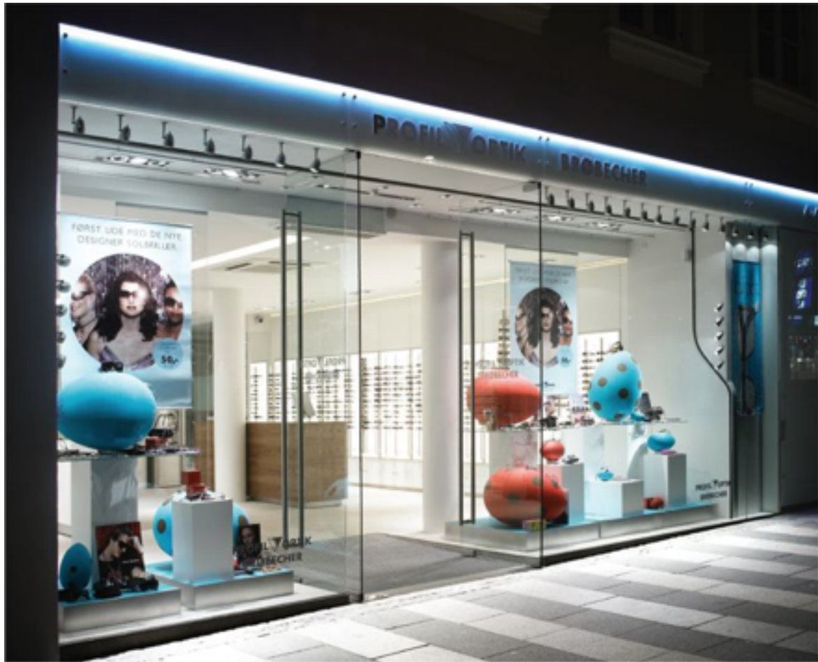
Figure 6.8 A typical straight front façade with display windows flanking the entrance to either side. Also, this is a rather typical mall shop front, with an all-glass façade, floor-to-ceiling glass panels, and no bulkhead. Merchandise needs to be raised up off the floor with risers or on platforms.
